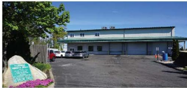
Neat and Clean Facility
