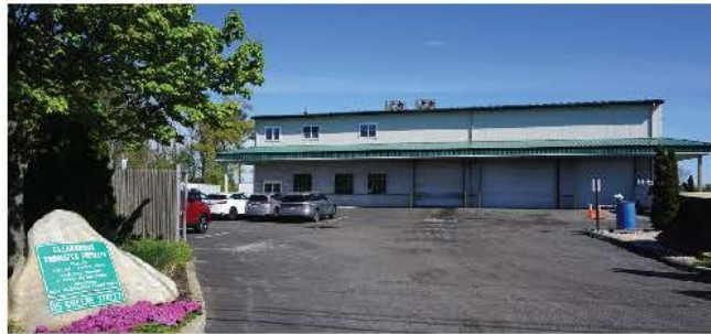
Neat and Clean Facility
