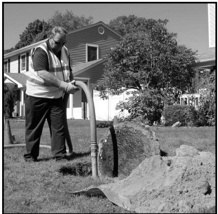
LILWA answers septic system inspection questions and demonstrates proper servicing
