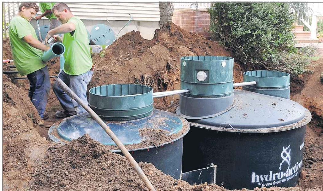
Suffolk County seeks to motivate 360,000 homeowners in unsewered areas to install cleaner systems.
